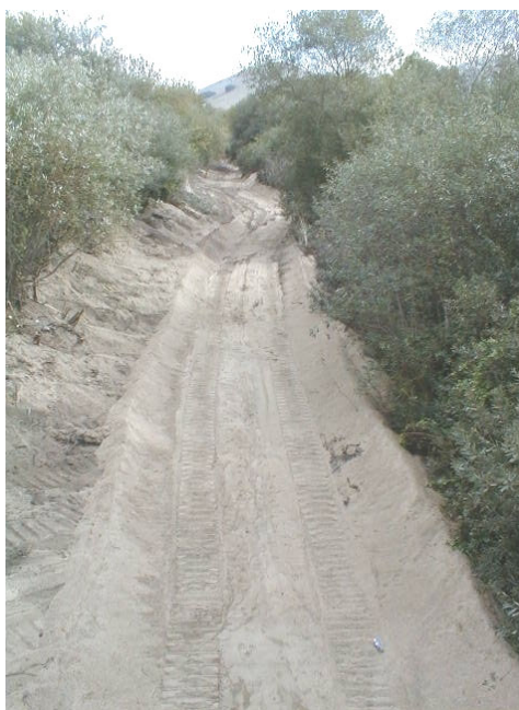
Figure 7.9. Bulldozing of the creek channel between GAB-HER and GAB-CRA, Aug 2000. Photo: Joel Casagrande.
