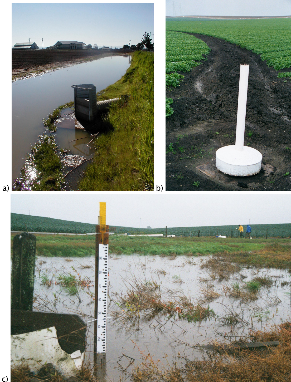
Figure 7.25. A selection of on-farm measures for runoff control: (a) a typical detention basin with standpipe and outlet pipe, (b) a catch basin that can easily be manually excavated at regular intervals, (c) a broad vegetated area that intercepts and diffuses runoff from a small agricultural watershed. Photos: a) Don Kozlowski, Feb 2001; b) Fred Watson, 3 Oct 2001; c) Fred Watson, 24 Nov 2001.
