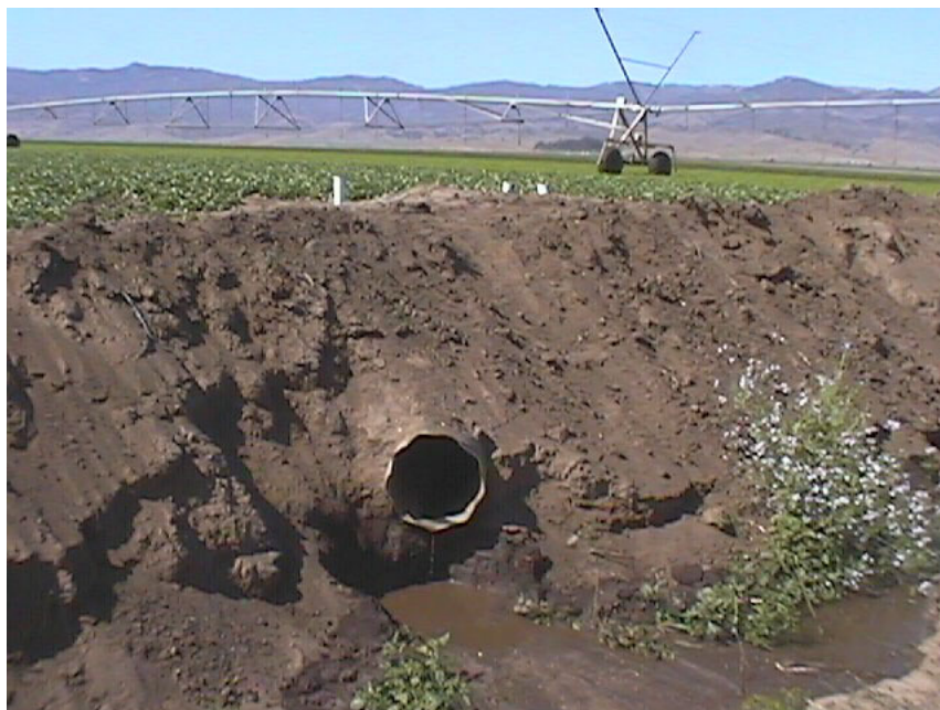
Figure 7.20a. Pipe used as sampling point draining field under linear irrigation. Photo: CCoWS, Summer 2000.
