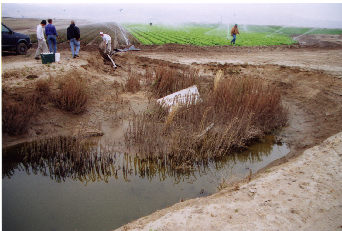
Figure 7.16. Monitoring runoff entering an on-farm sediment detention basin. Photo: Fred Watson, 30 June 2000.
