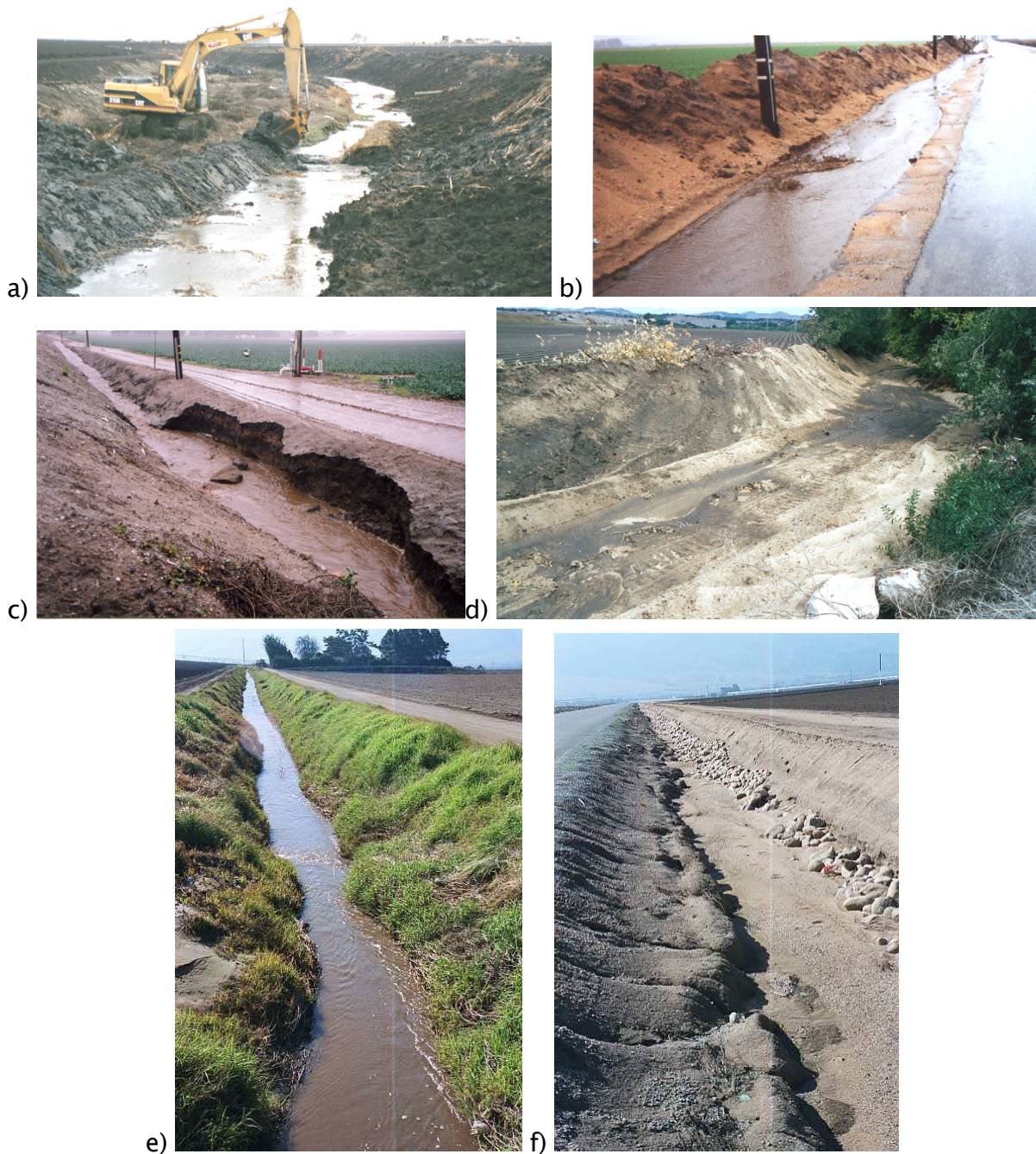
Figure 7.26. Sediment delivery ratio of agricultural ditches and streams: (a), (b) less than 100% delivery in excavated ditches, (c) greater than 100% delivery in an eroding ditch, (d) uncertain delivery ratio in a stream with riparian bank vegetation removed, (e) bank stabilisation along a grassed ditch, and (f) limited sediment retention in a cobbled ditch. Photos: Fred Watson: a) Jan 2001; b) 11 Feb 2000; c) 11 Feb 2000; d) Oct 2000; e) Feb 2002; f) Feb 2002.
