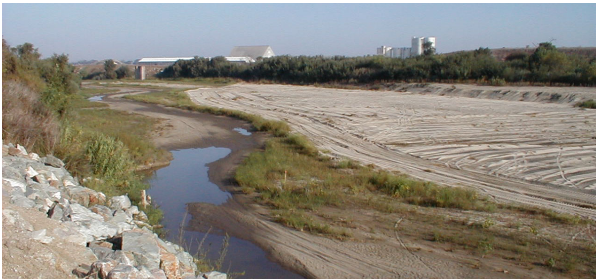
Figure 5.12. Channel grading and vegetation removal for flood control – Salinas River at Spreckels. Photo: Thor Anderson, Fall 2000.
