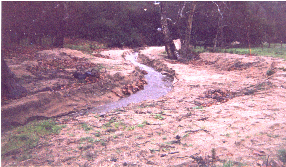
Figure 6.15. Recent floodplain deposition of sediment below the headwaters of Chualar Canyon, and subsequent channel maintenance using earth-moving equipment. Photo: Fred Watson, 2000.
